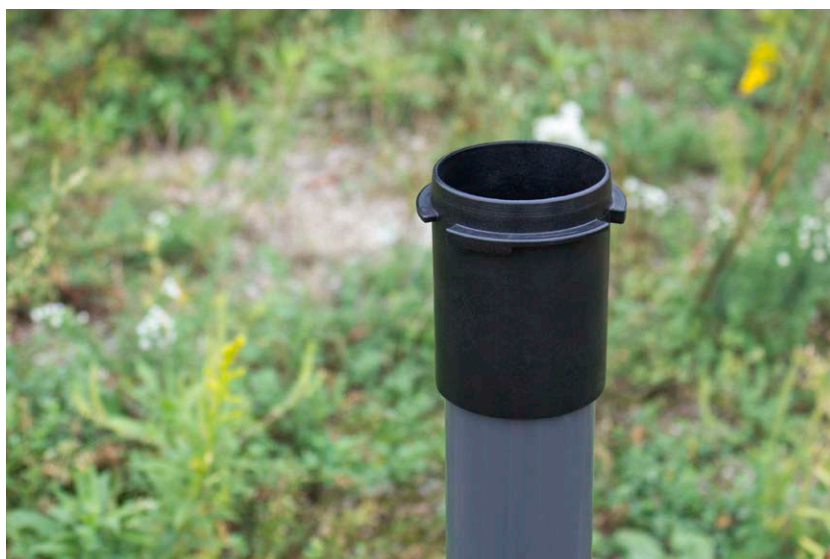
Figure 6-3 Install the Well Cap Base
