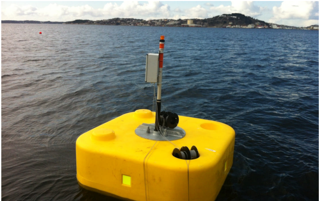
Fig. 6 – Remote read-out solution example: Monitoring of the seabed close to a sea-port building site. A telematics gateway is installed on buoy for communication via the mobile phone network. Set thresholds and get alarms as e-mail or text messages to your phone.
